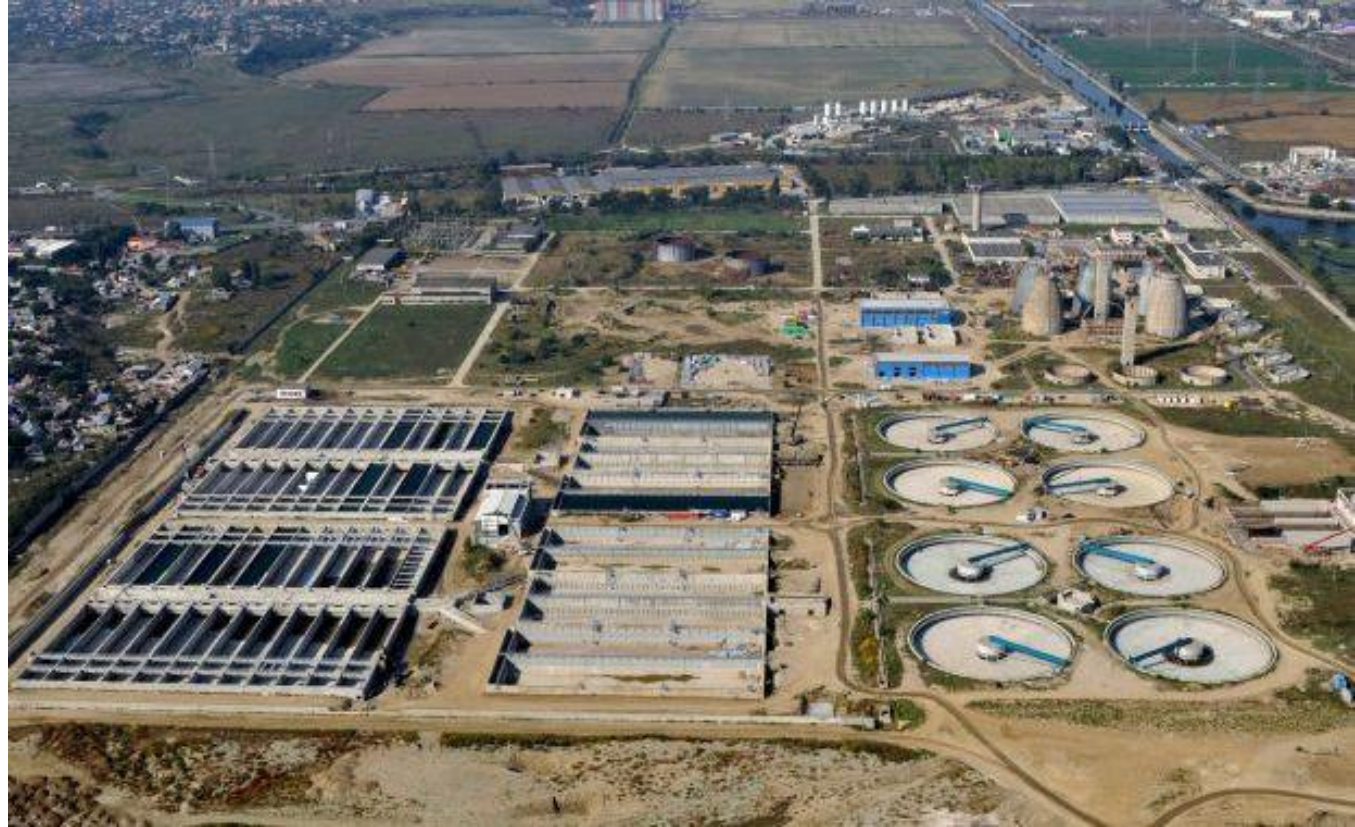
Glina Wastewater Treatment Plant
