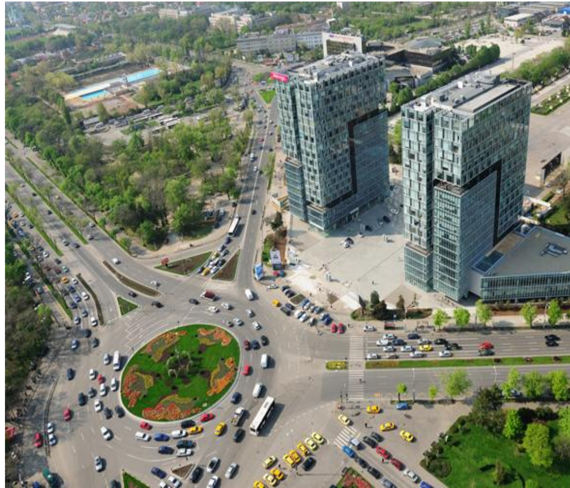
City Gate Towers, Bucharest
